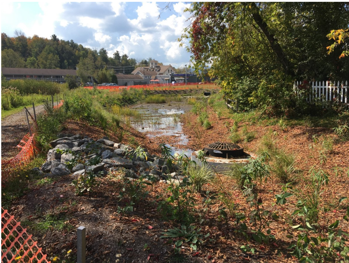
Figure 16. Picture of a stormwater treatment wetland installed in the Town of Brighton.
