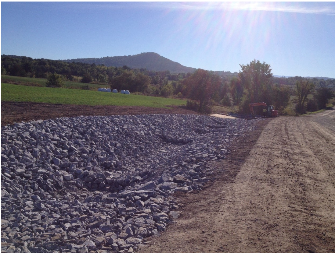
Figure 9. Thompsons Point Road, Charlotte road ditch with check dams and bioretention basin
