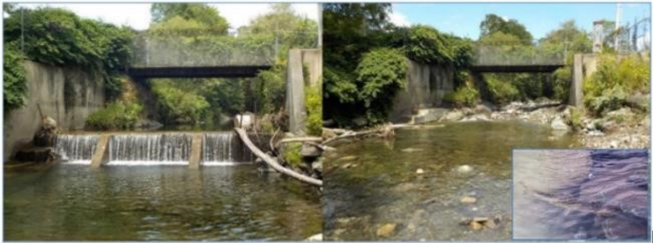
Figure 14. Before and after photos of the Geer Dam removal on the Ompompanoosuc River. Inset photo of a Brook Trout waiting near the dam face during the removal.
